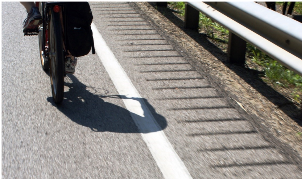
Continuous shoulder rumble strip along KY 11 in Slade
